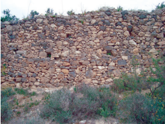
Fig. 3 Dilapidated, circular bee-garden (melissokepos) built with walls of loose stones and holes. Unpublished bee-garden (circa 17th - 18th c.) in the place named Melissokepos from Gouves Pediados, Irakleion Crete (Photo Ilias Anagnostakis).
