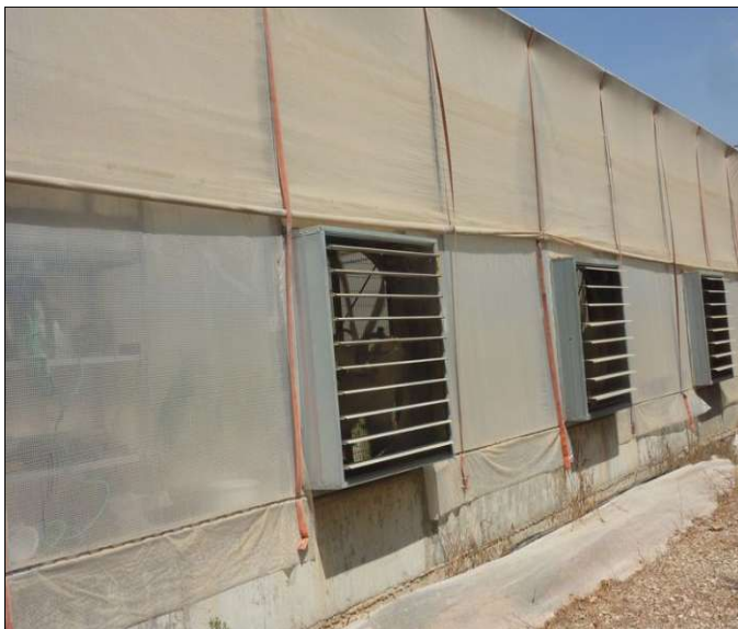
Fig. 18. Greenhouse ventilation system.
