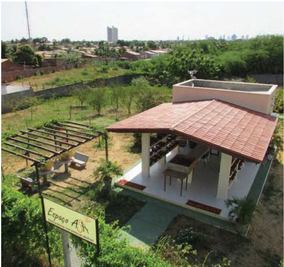
Figure 2. Facility designed to house palynology laboratory, stingless bee hives and a bee garden (Espaço ASA) at the Federal Rural University of the Semi-Arid, Rio Grande do Norte, Brazil (Universidade Federal Rural do Semi-Árido, UFERSA).
